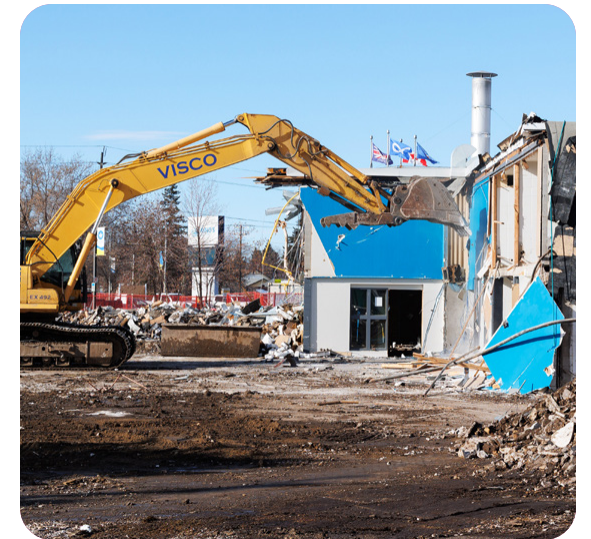
Admin building and Level Coffeeshouse demolition
